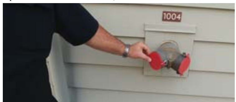
Aubert tests the fire department connection.
